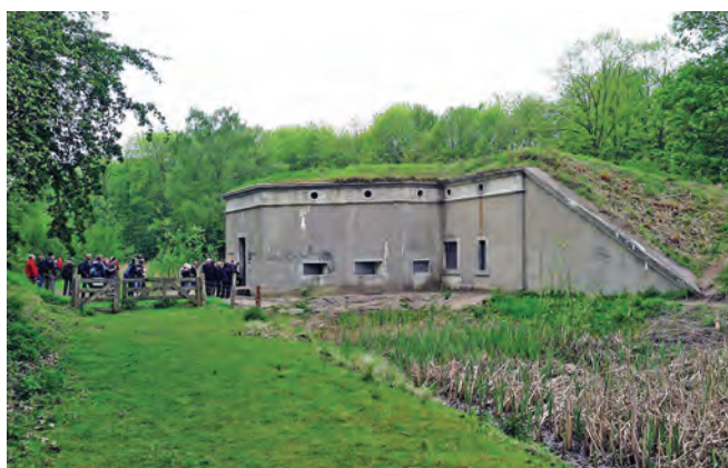
Twin Caponier within the moat of Vestvolden. The second opening from the right is where the searchlight would have emerged from on overhead rails to illuminate the moat
